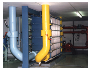
Plate type Heat Exchanger
